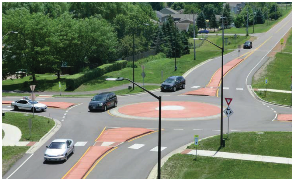
Example of a single-lane roundabout. Source: FHWA
